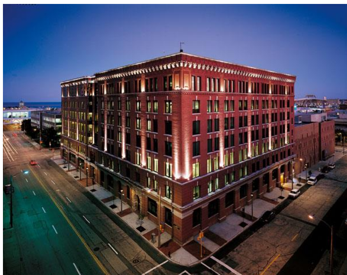
Obr. 7.14 Brengelovo centrum v USA, Milwaukee
